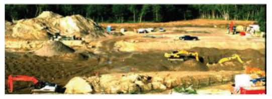
Picture 1 - Excavation through natural liquefiable deposit
