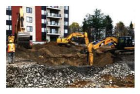
Picture 5 - Exposed steep excavation face in earlier conditioned soil
